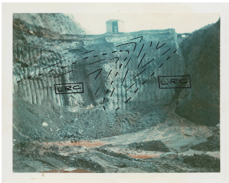
Figure 7 Some of the images in the MSARS archive were used as working tools to identify geological formations in preparation for mining activities. This photo includes notations regarding rock shape and lines that will be used for further geological interventions. (Image author unknown).
